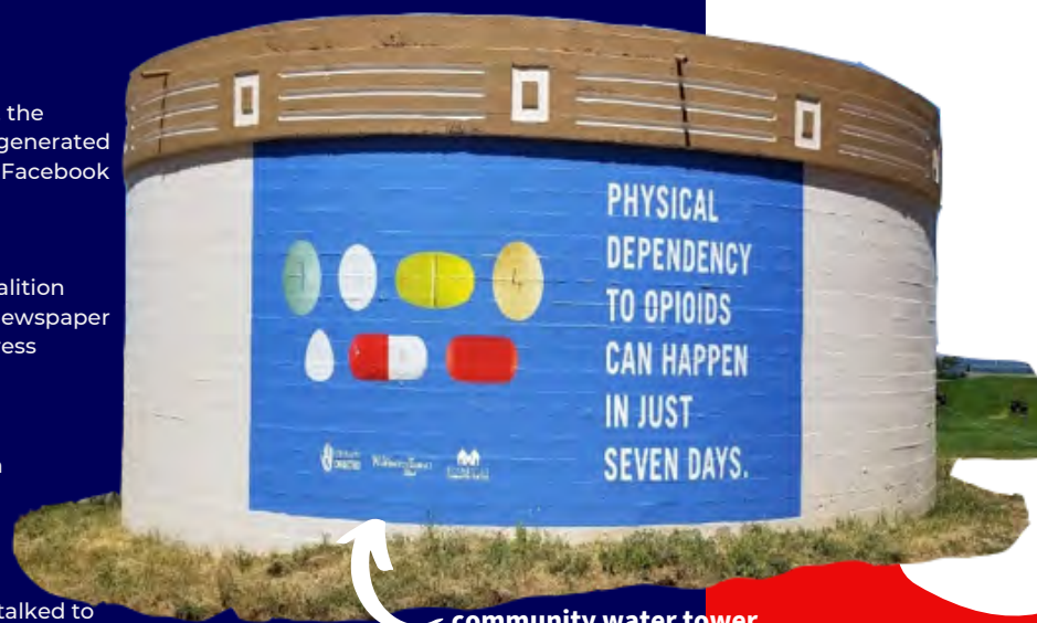
community water tower
